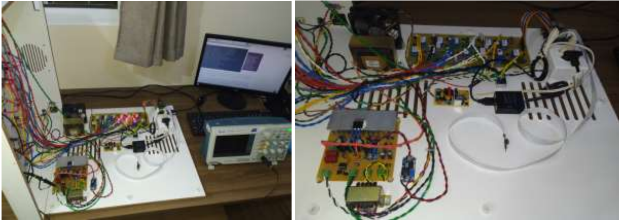
Figure 15. Testing of components (A) GPIO and PWM measurements (B) Open cabinet.
