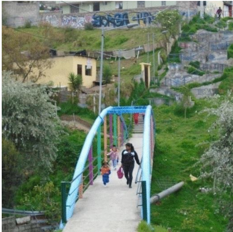
Figure 2. Bridge over restored ravine “Habas Corral” in “La Pulida”.
