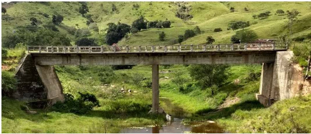
Figure 3. Bridge in the city of Correntes-PE.
