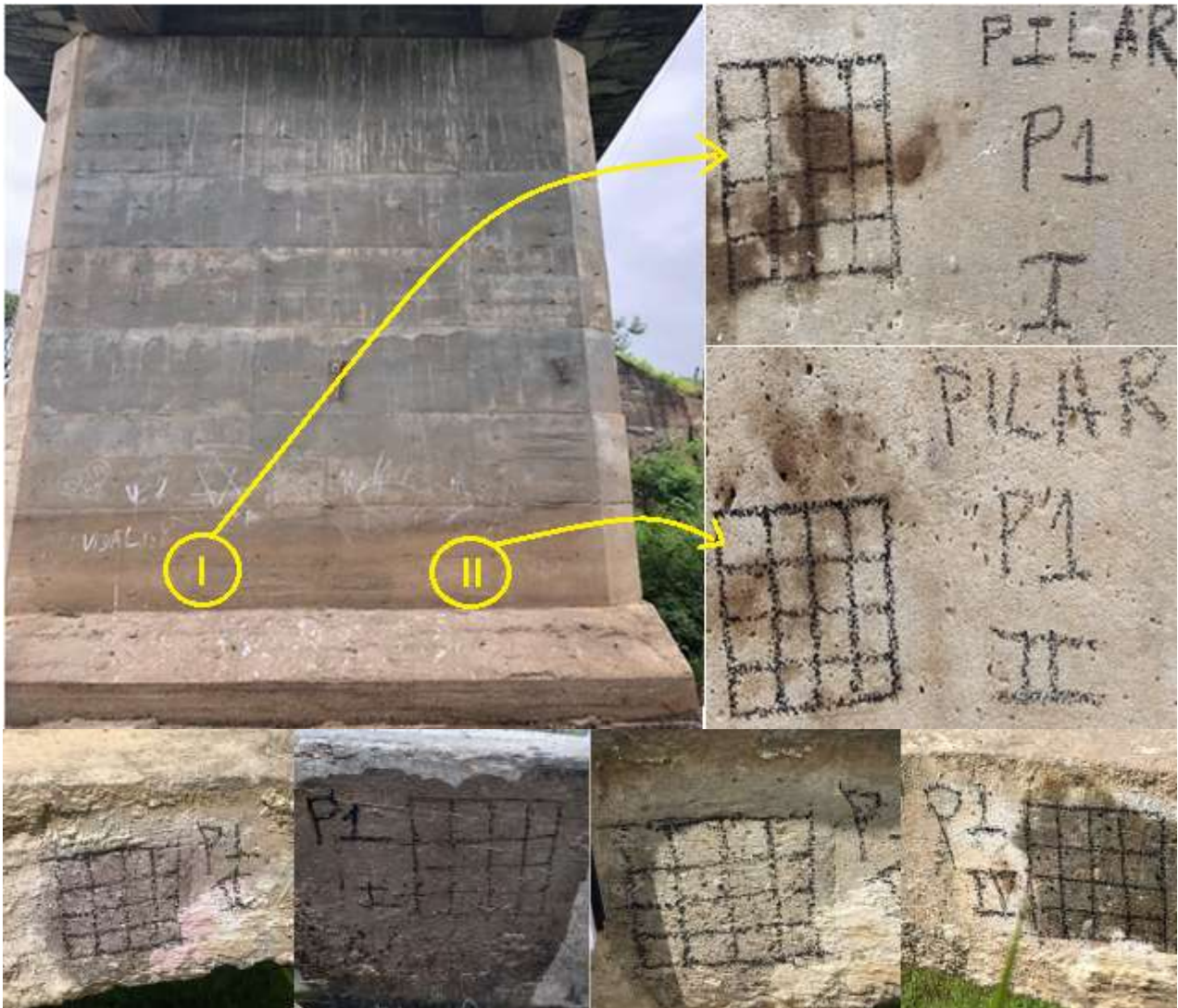
Figure 4. Conducting sclerometry tests on the catwalks and central pillar.
