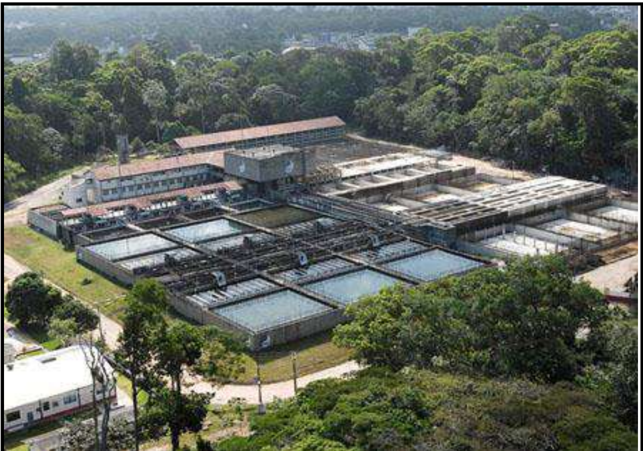
Figure 3: COSANPA Treatment Plant within the limits of the PEUT
