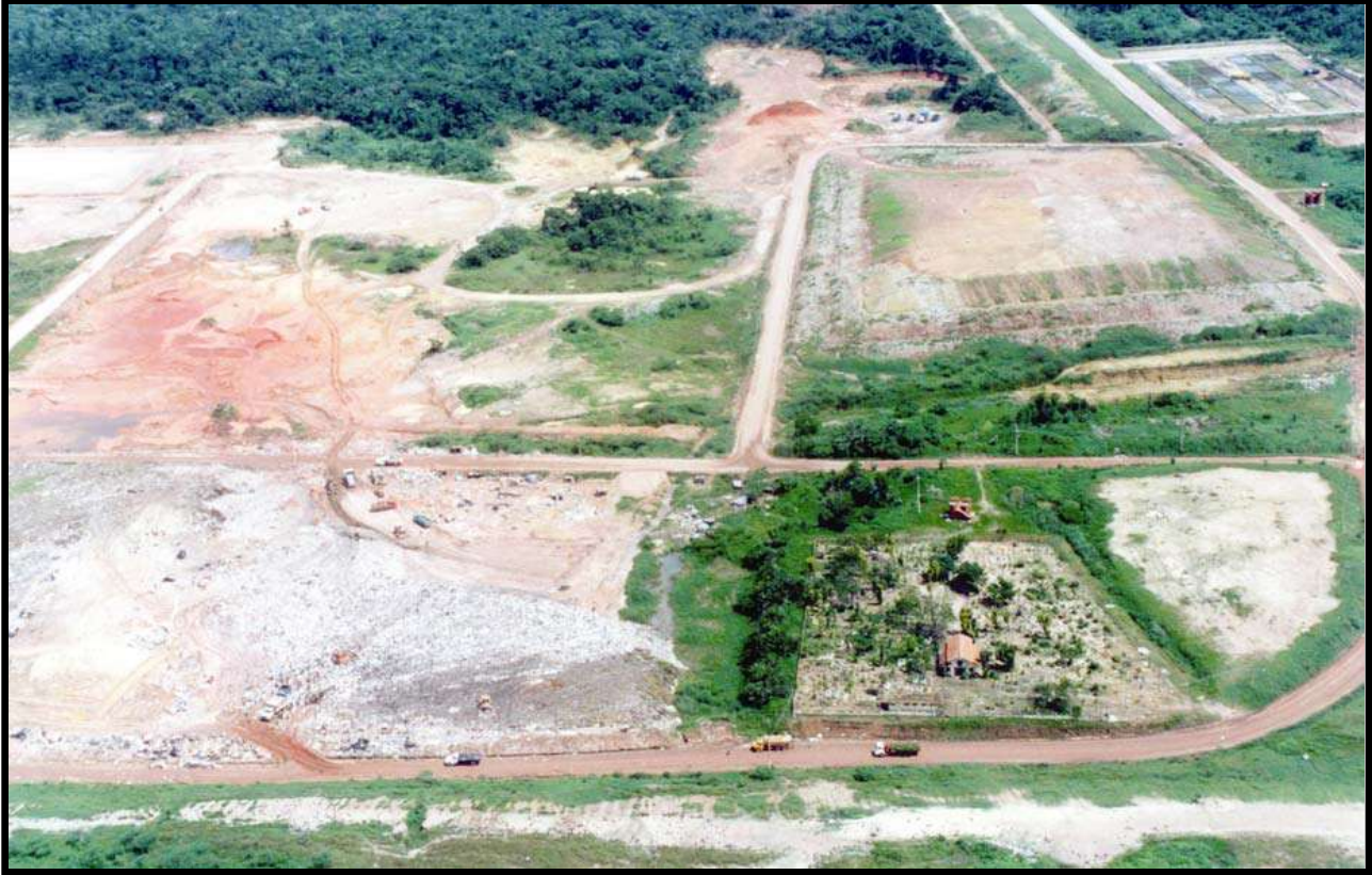
Figure 2: Aurá embankment in the area surrounding the PEUT
