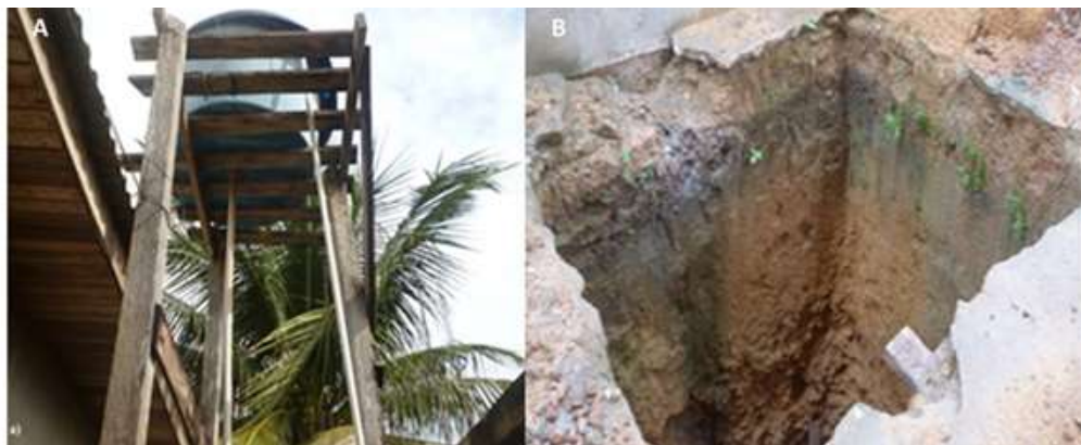
Figure 4. Water and sewage system-a) water box for storing water collected from underground aquifers, b) septic tank construction.
