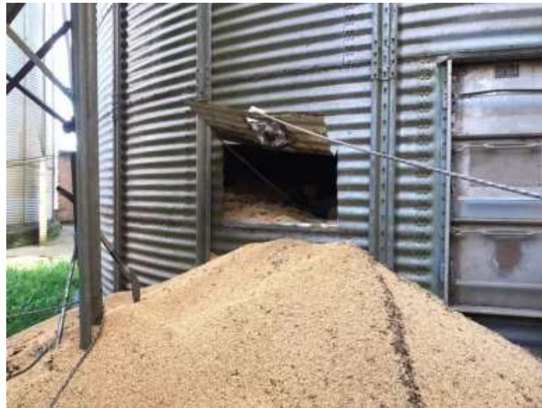
Figure 6. Detail of the opening at the bottom of the structure for removing soybeans and rescuing the victim.
