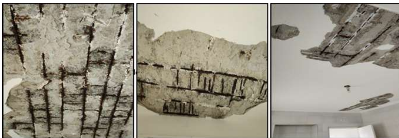
Figure 3: Reinforced concrete slab of the building.
