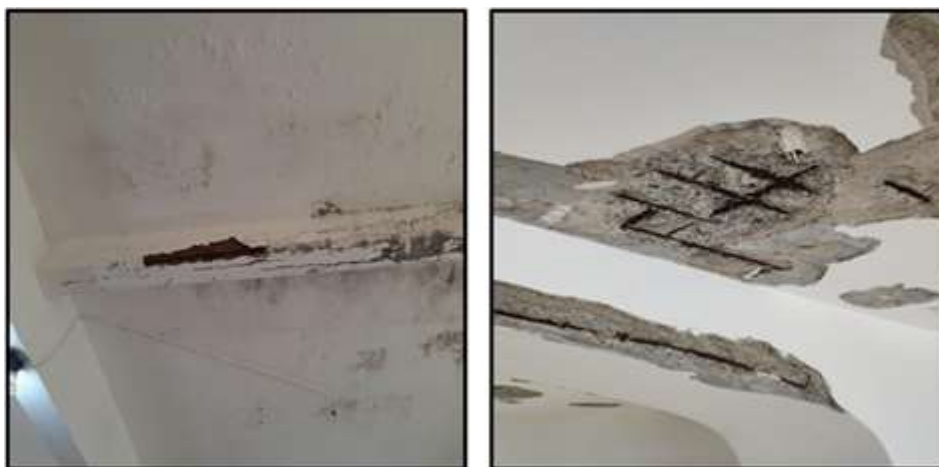
Figure 4: Reinforced concrete beams of the building.
