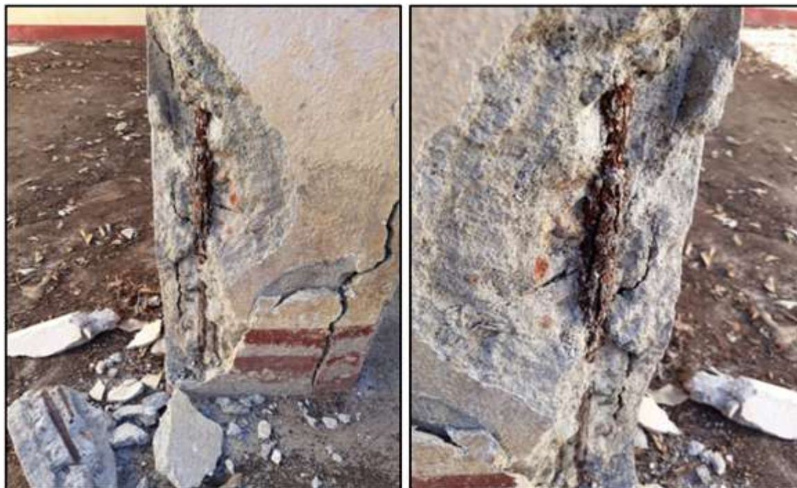
Figure 2: Reinforced concrete column on the ground floor of the building.
