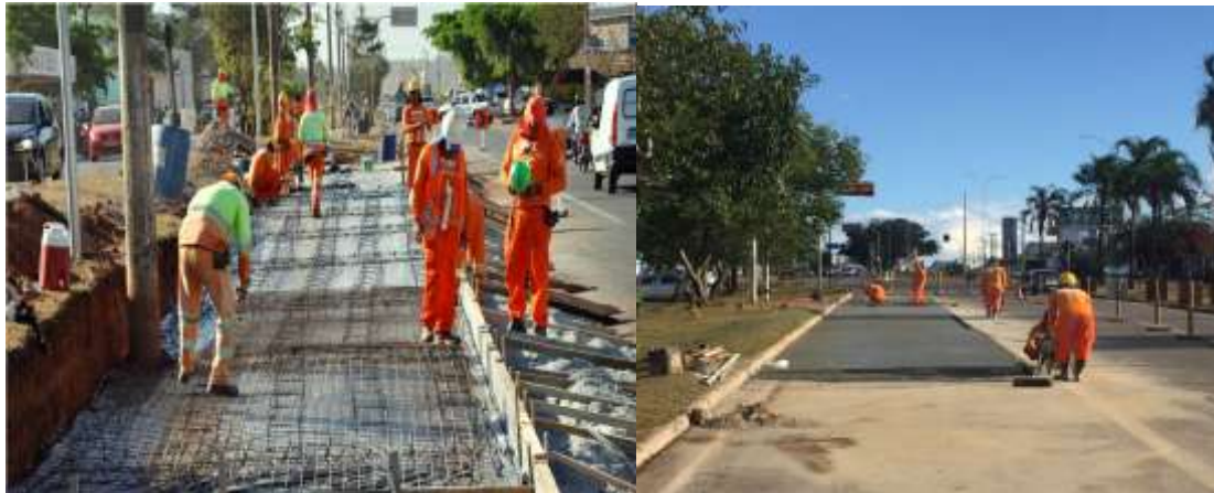
Figure 2 - Preparation of the PCC slabs.
