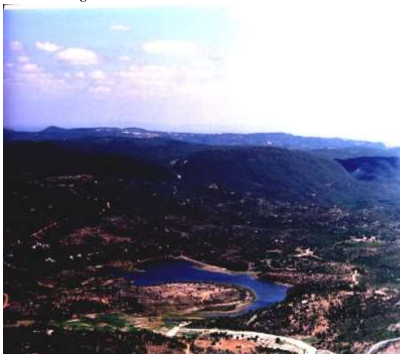
Figure 2: Aerial view of the Mamao Reservoir.
