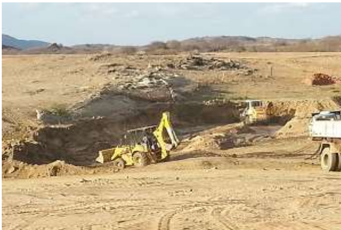
Figure 3: Backhoe and shovel filling machine removing sediment from the weir bed.
