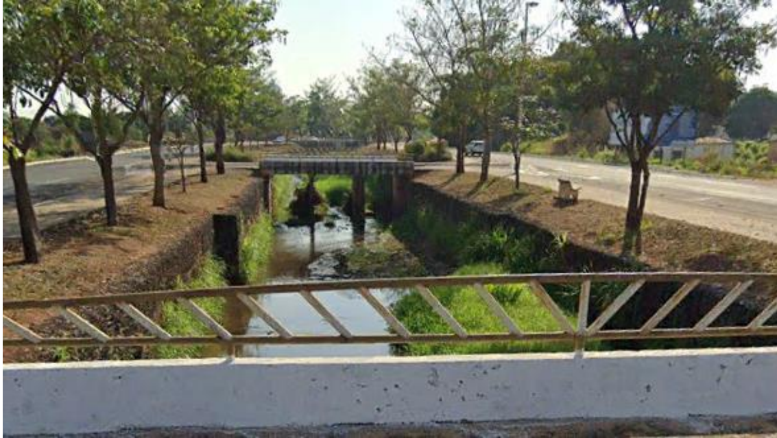
Figure 2 - Neblina brook, in an area where it is channeled and receives a large effluent load, before point 06.
