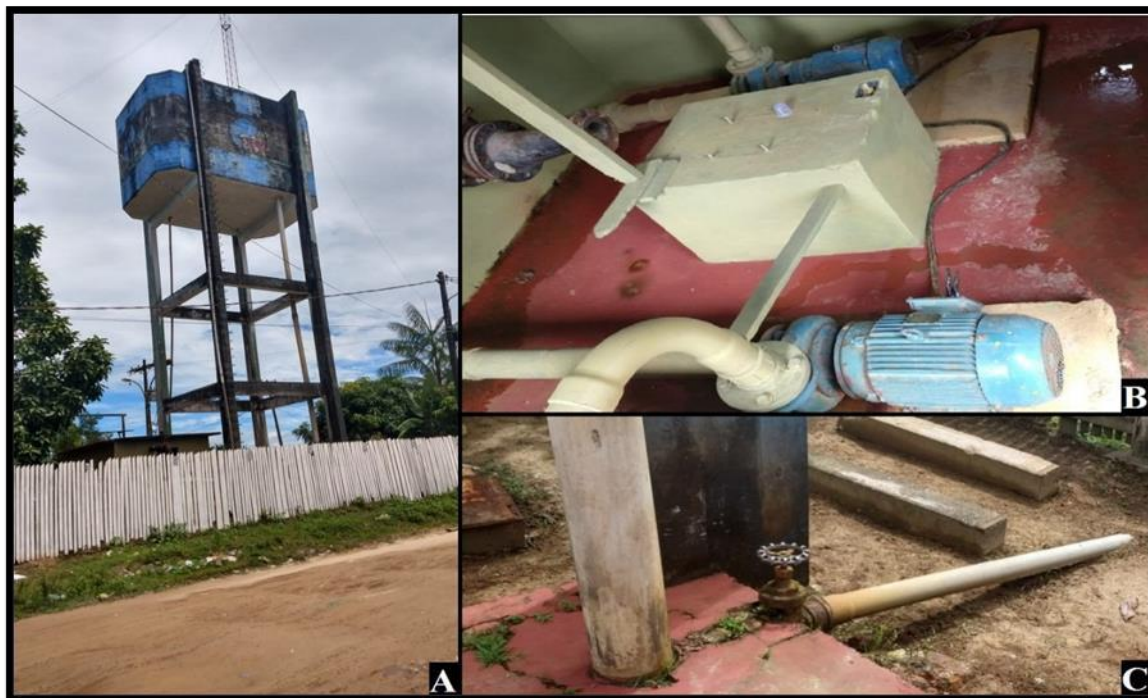
Figure 7 - A: Water reservoir; B: Pumps for pushing water into the reservoir; C: Water outlet valve for the consumer.
