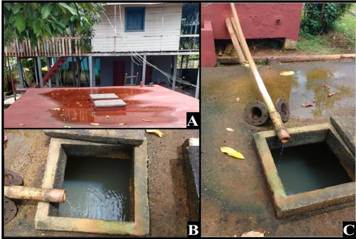
Figure 6 - A: Cistern; B: Interior of the supplied cistern; C: Plumbing coming from the filter to supply the cistern.
