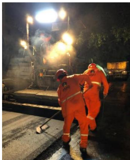
Figure 5 - The laborers distributing and leveling the asphalt mix.
