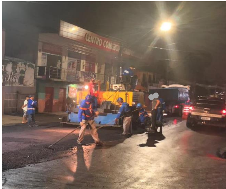
Figure 6 - Car driving alongside the workers who are working on the stretch.
