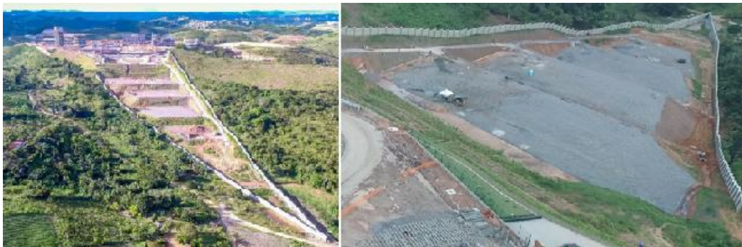
Figure 2 - Installation location of the UACSA photovoltaic plant.
