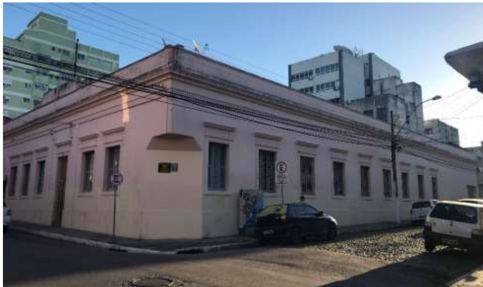
Figure 6: 2 Facade of Block 2.10 Street Félix da Cunha, 821.
